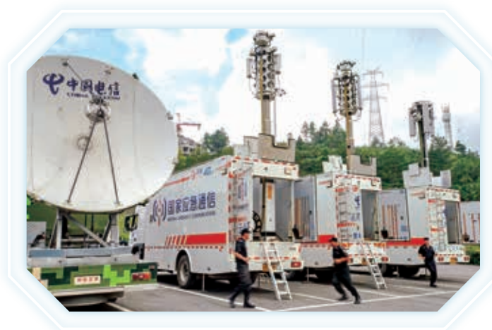
Demonstration of 5G emergency telecommunication assurance
