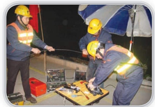
Access lines disaster relief technicians urgently spliced optic fibre cables
