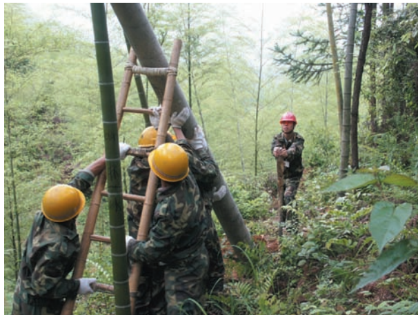
China Telecom workers were constructing networks in rural village area
